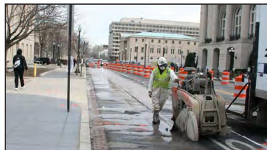
*A construction worker makes the first cut in the asphalt of E St. NW that commences work on the Museum. The Museum will be located underground on the south side of E St. (the right side of the picture) between the building with the columns and the building with the green roof.*
